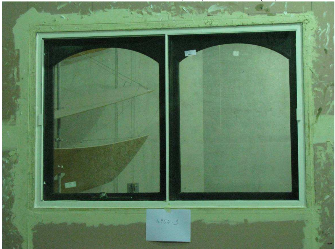
Figure 1. Installation of combined Secondary Window System (Receive Room Side)
